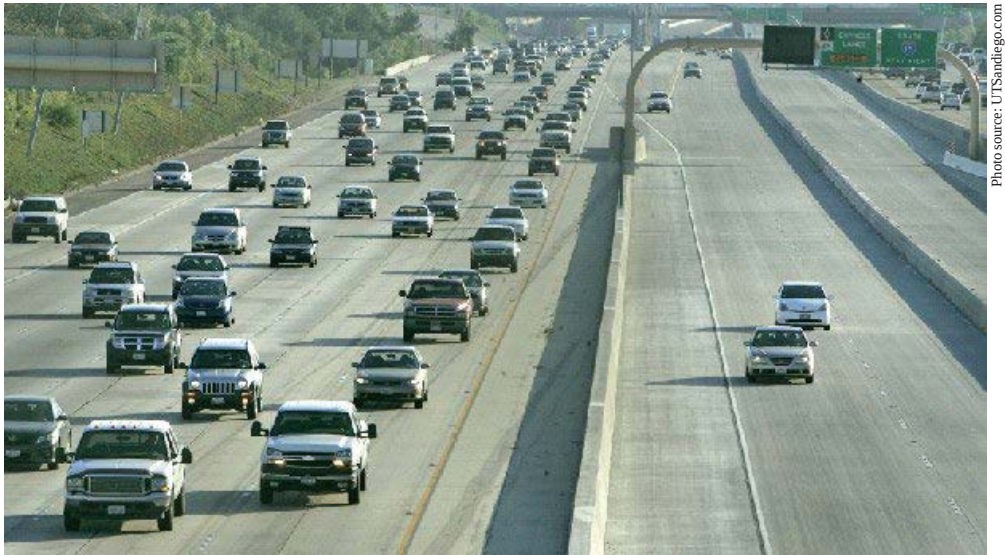
Figure 13. Photo. I-15 Express Lanes in California.
