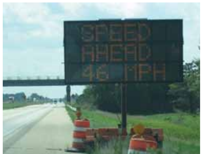
Figure 22. PCMS messages were modified from a generic message (left) as stated in the contract to a more specific message (right).
